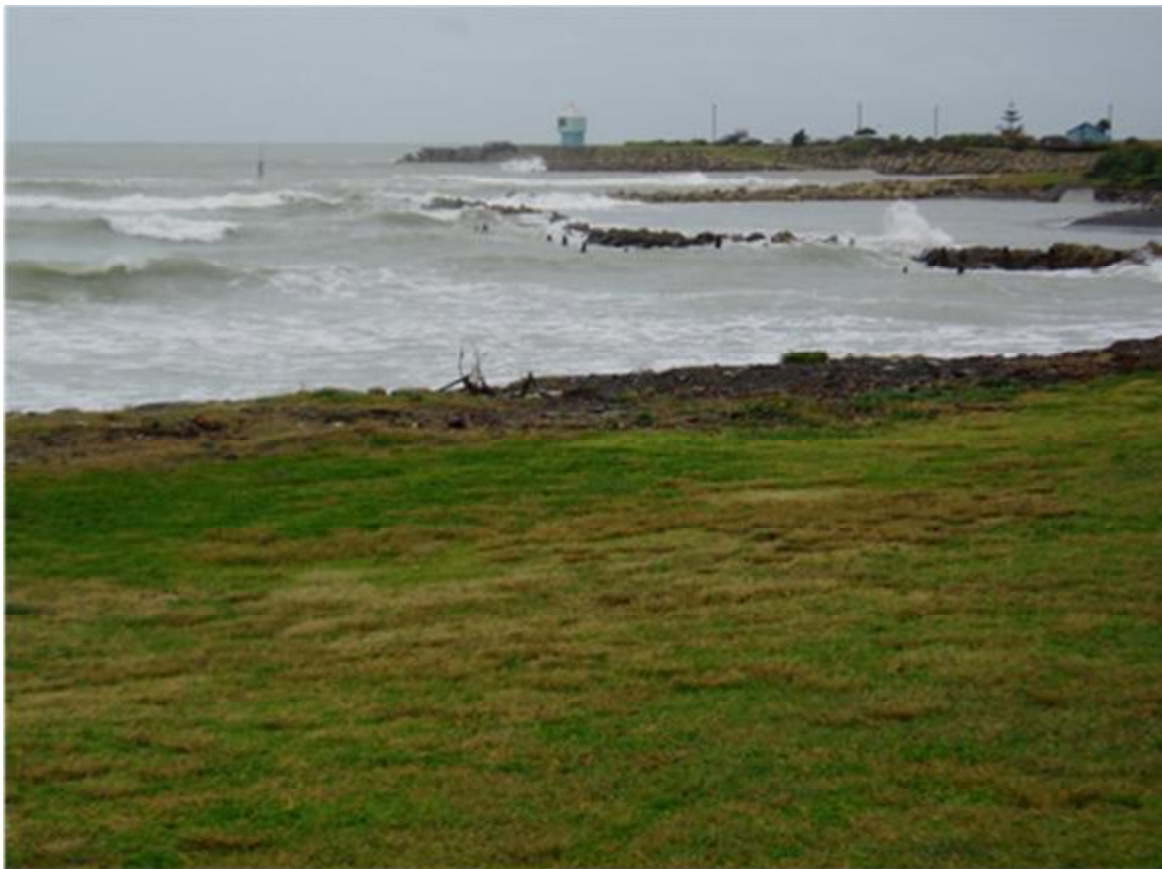
Photo 2: Existing Wall/Breakwater during Sea Storm
