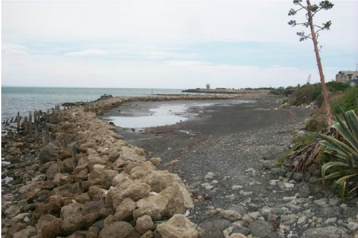
Photo 1: Existing Wall/Breakwater at Low Tide
